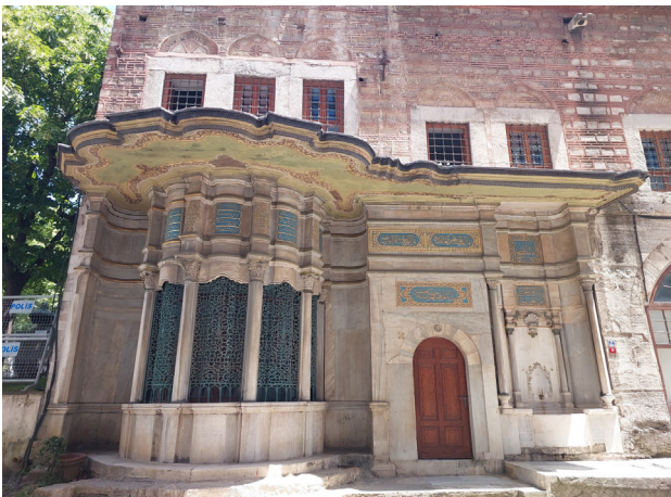
Seyyid Hasan Paşa Sebil and Fountain.
